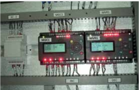
MIACs used to control a mid scale hydroelectric power station in Sri Lanka.
